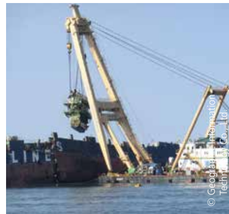
Removal of the engine
