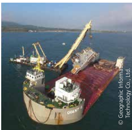
Removal of living quarters
