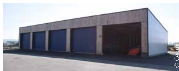
Cedre's storehouse completed
