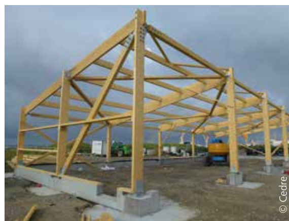
Cedre's storehouse under construction
